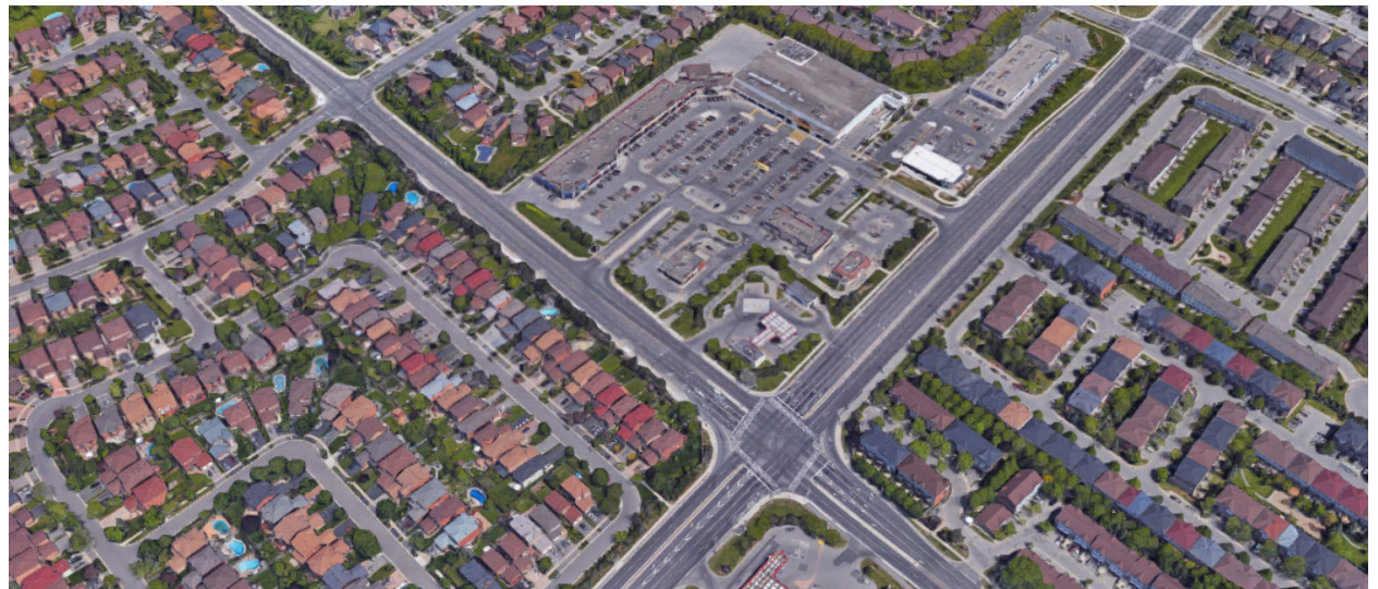
The intersection of Creditview and Britannia: The commercial plaza and large parking lot at the northeast corner of this intersection offers a large site with redevelopment potential.
